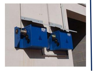
Avoid fixing the motor in a damp place or where there is the possibility of pouring any liquid onto it. If it cannot be avoided, protect it as much as possible (with an awning, or with some additional protective housing, for example)
